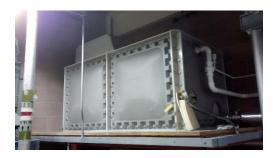
Further to the new sectional tank being erected, DMA Canyon plumbing experts removed the temporary mains bypass and plumbed in the new tank to the building's water system. Once installed, the tank and associated hot and cold water system were disinfected in accordance with BSEN 806 and ACOP L8 with certification provided to the client.
